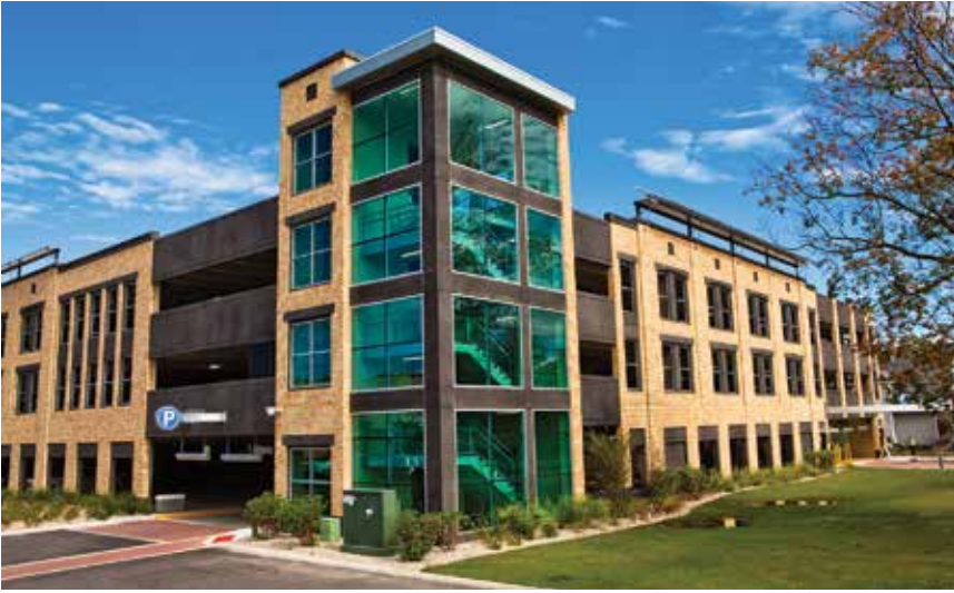
The Old Town Parking Structure in Traverse City, Mich., features a variety of sustainable-design concepts generated from public design charrettes. These include a green roof over a portion of the roof-level parking and atop the stair towers, charging stations for electric vehicles, solar panels to generate electricity, and a snow-melt system.
