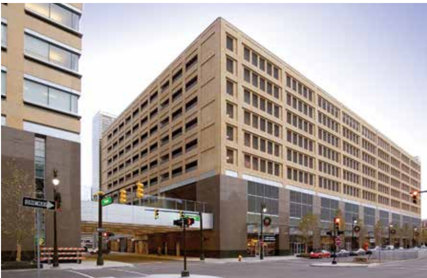
The Campus Martius One parking structure in Detroit, Mich., was value-engineered from cast-in-place to precast concrete to provide a more efficient design. The nine-story, 2,100-car structure features a façade clad with Mankato limestone to match a nearby office building and 16,000 square feet of ground-floor retail space.
